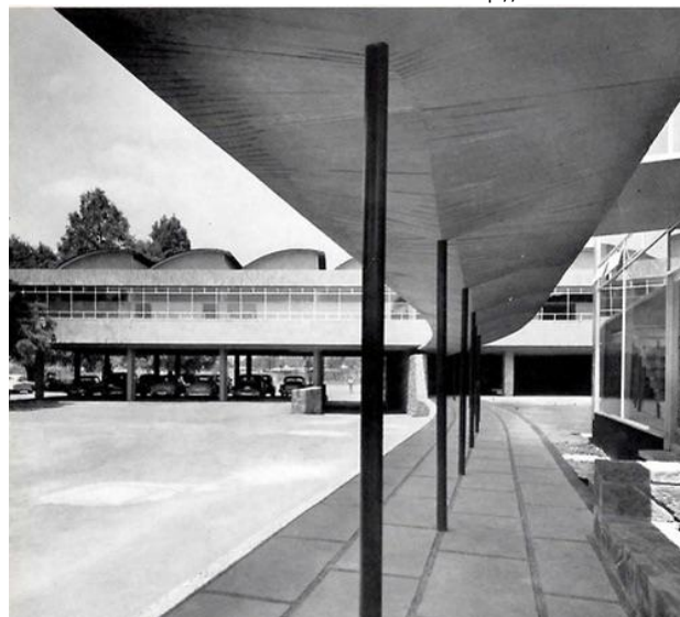
Figure 6. Interior view of the courtyard between production and storage in the CIBA Laboratories, Churubusco, Mexico 1954. Alejandro Prieto, assistant architect: Enrique Manzaneres and technical assistant: Félix Candela. http://www.tumblr.com
