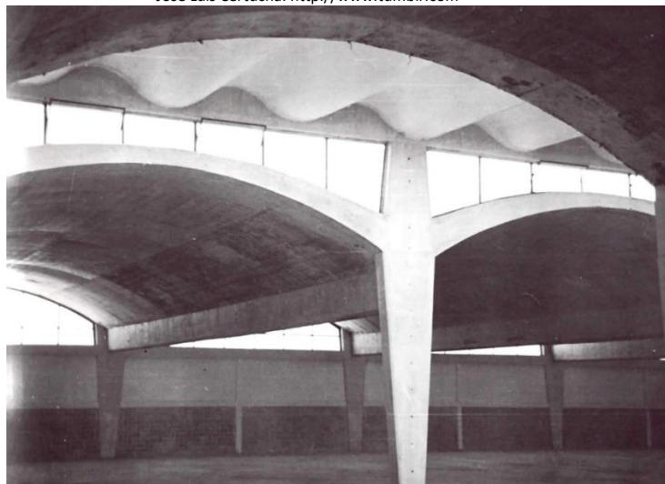
Figure 2. Interior view of the Pisa Warehouse, San Bartolo, State of Mexico, Mexico 1951. Félix Candela and José Luis Certucha. http://www.tumblr.com
