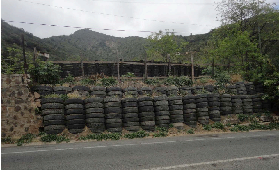
Figure 6. Medialuna retaining wall of "La Dormida", Olmué. (Photo: Gustavo Sarabia)
