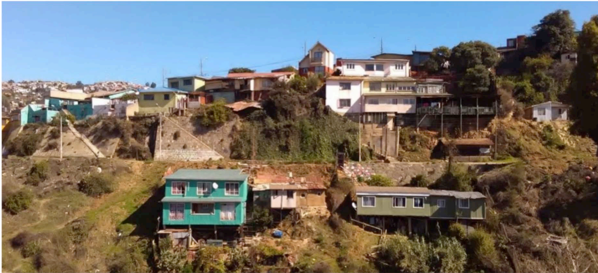
Figure 2. Houses on land contained by walls and others on pillars, Valparaíso. (Source: unknown)
