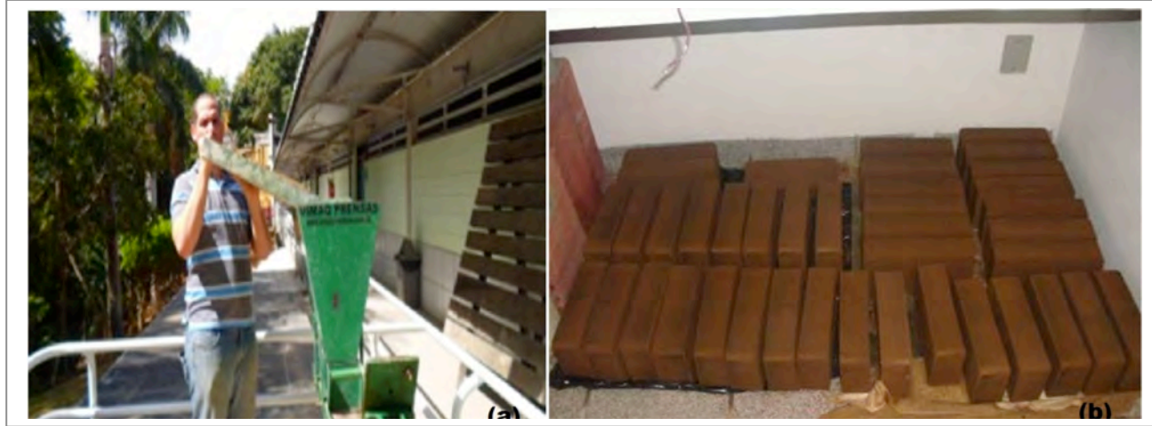
Figure 3. a) Block pressing; b) Curing of soil-cement blocks
