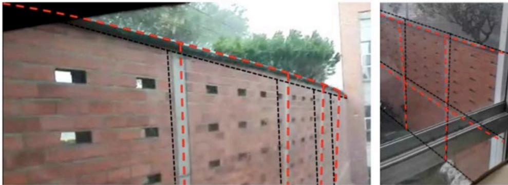
**Figure 5.** Wall deformation at incipient collapse seen from two different views (black thin lines indicate original at-rest position. Red discontinuous lines indicate deformed shape at incipient collapse)
