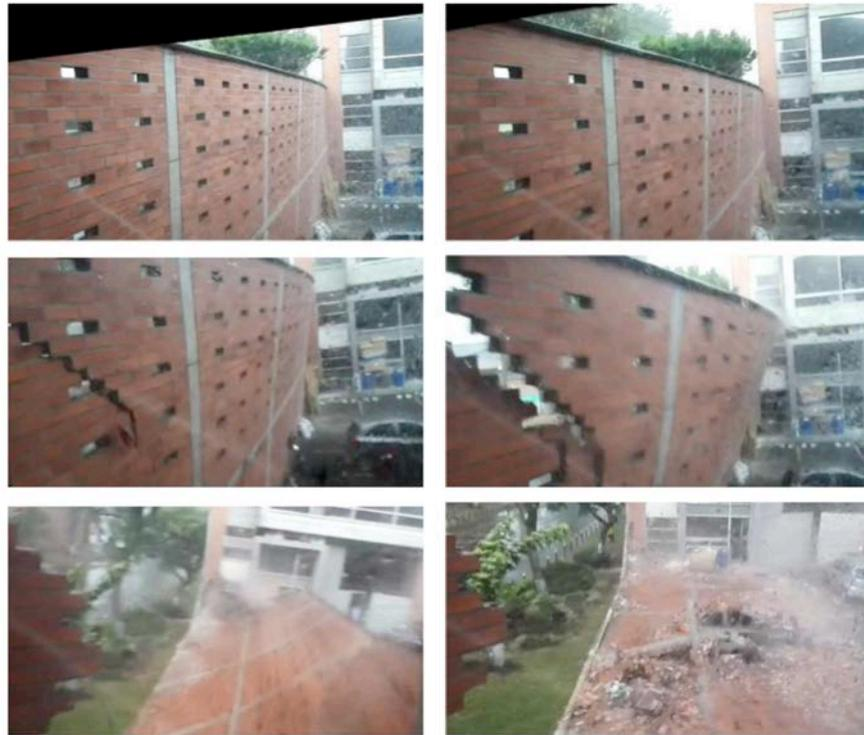
Figure 2. Collapse sequence
