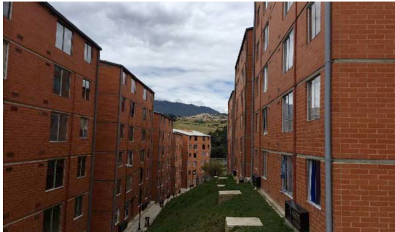
Figure 1. Interior view of the project
