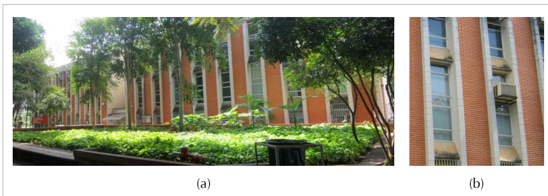
Figure 1. Entrance of the building (Southwest) (a) and detail of the facade(b)
