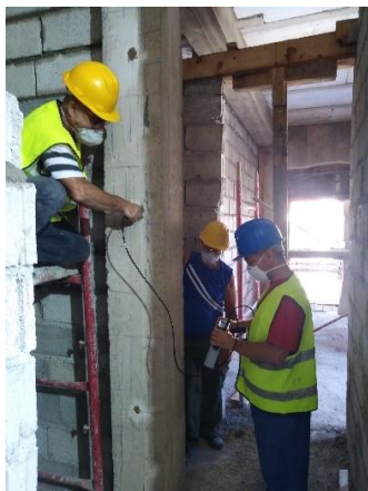
Figure 1. Undergoing of measurements on a column
